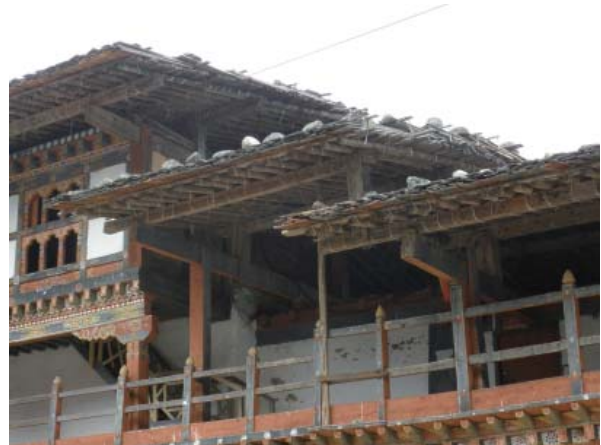
Photo 2-4-5 Single roof with stones on top.
