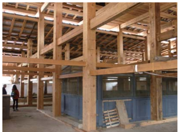
Photo 2-2-6 Reconstructed roof structure on top of Utse.
