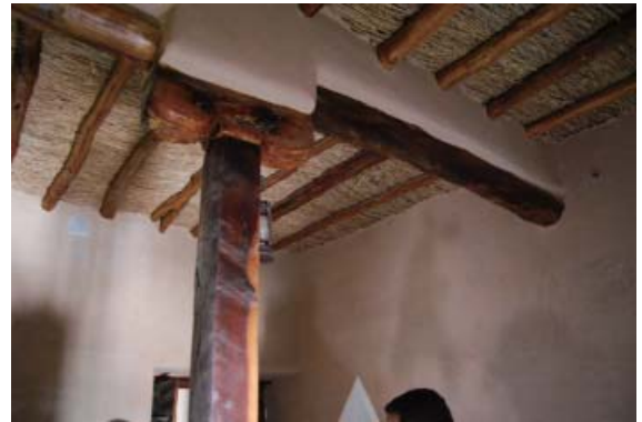
Fig. 14-7 The ceiling, supported by a bracket and beam atop the column.
