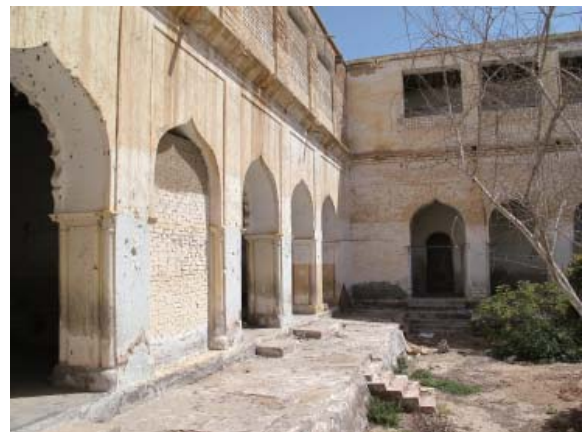
Fig. 11-6 A series of ogee arches around the corridor enclosing the courtyard.
