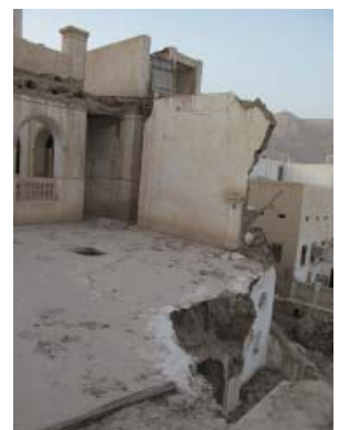
Fig. 9-7 The collapsed part of the terrace.
