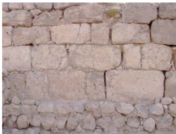
Fig. 1-4 Rectangular ashlar masonry.
