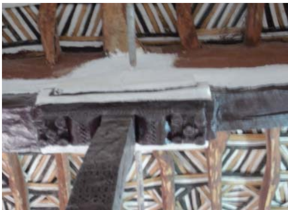
Fig. 16-5 The frame of the ceiling, and the bracket.
