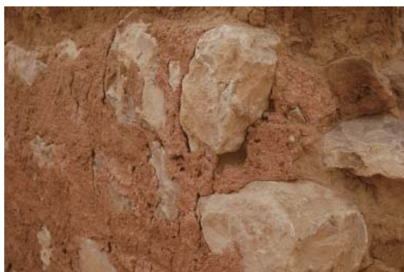
Fig. 2-4 Split stones embedded on a wall.
