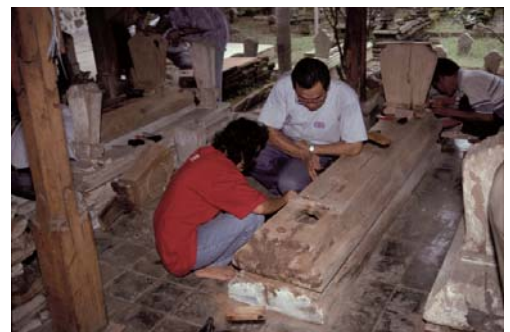
Training in ant repellent resin treatment using a wooden gravestone
