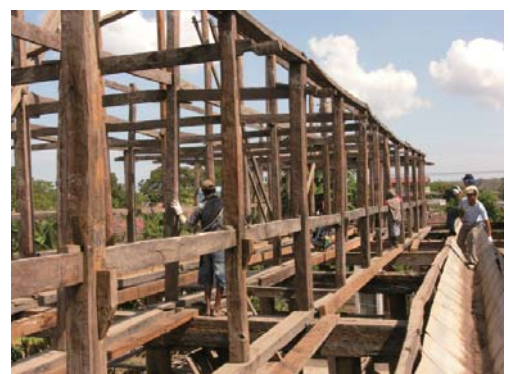
Repair of the roof truss
