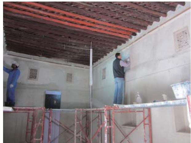
Fig.88 Restoration of interior decorations at Shaikh Salman House
