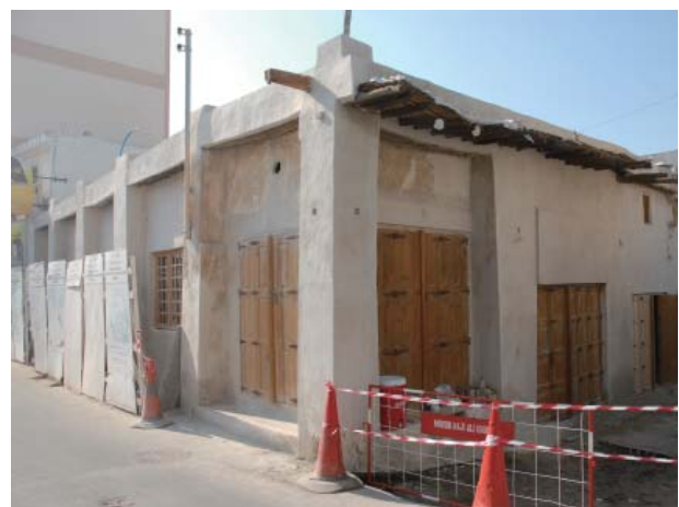
Fig.109 Renovation of a dukkan into a café
