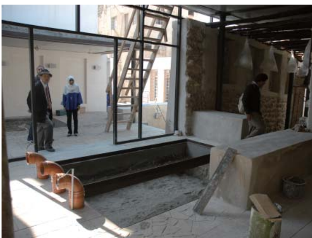
Fig.108 Renovation of a dukkan into a café
