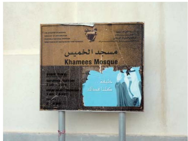
Fig.70 Faded information board
