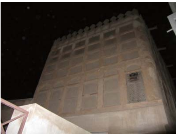
Fig.94 External view of Seyadi House
