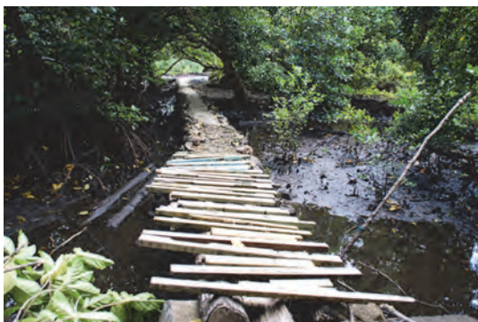
Photo 32 Accumulation of silt near a land bridge
