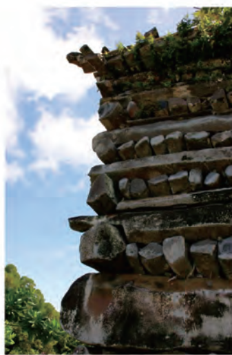
Photo 13 Northeast corner of the outer wall
