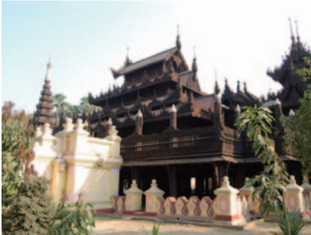
Fig.68 External view of Shwei-in-bin Monastery from the northwest
