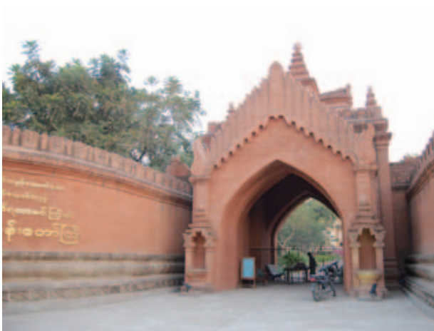
Fig.45 External view of the entrance to the Bagan Golden Palace and Palace Site Museum
