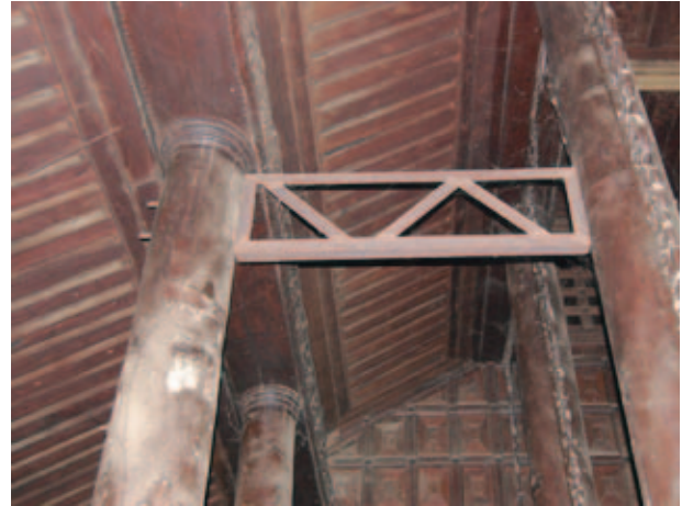
Fig.69 Steel truss beams installed in Shwei-in-bin Monastery for reinforcement
