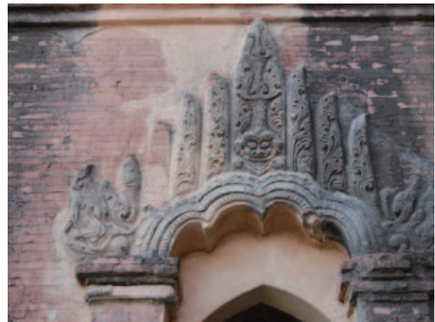
Fig.32 Close-up of the portion above a window at Dhamma-yan-gyi
