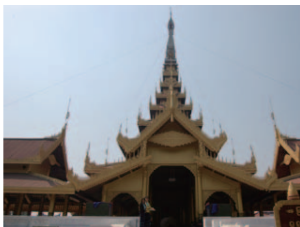
Fig.53 Central building in Mya-Nan-San-Kyaw Golden Palace
