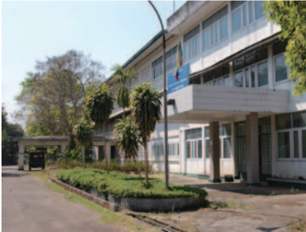
Fig.101 External view of the National Library
