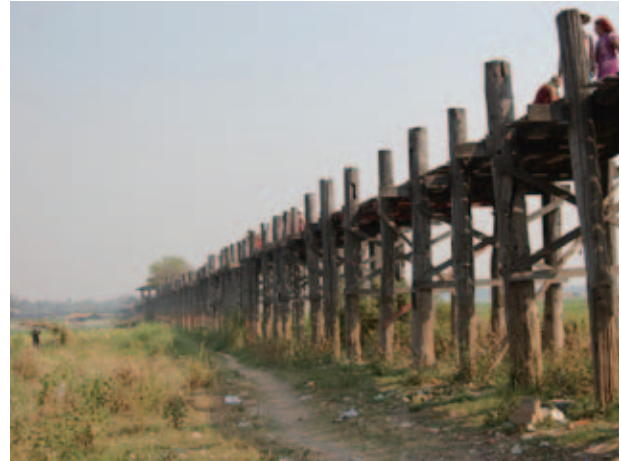
Fig.92 Close-up view of a bridge pier of U Bein Bridge
