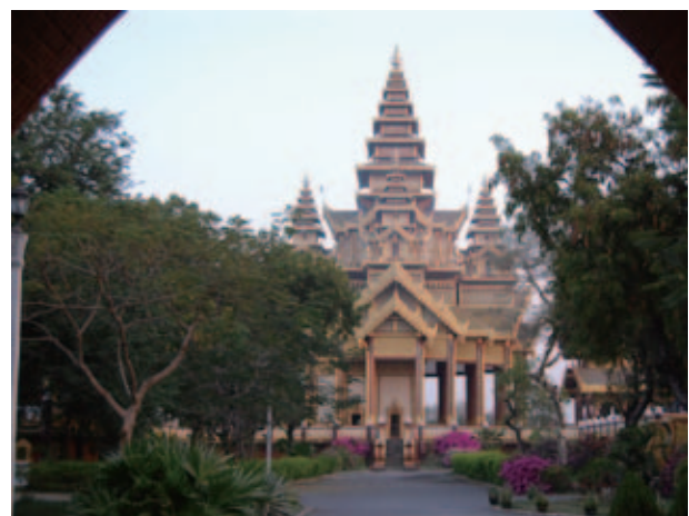
Fig.46 Main buildings of the Bagan Golden Palace and Palace Site Museum
