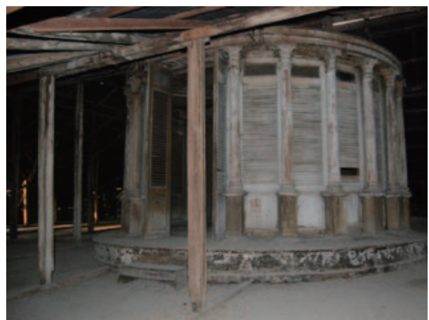
Fig.67 Inside of the attic of Thaka-wun Monastery
