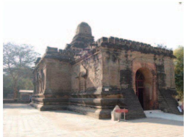
Fig.26 External view of Nan-hpaya from the southeast
