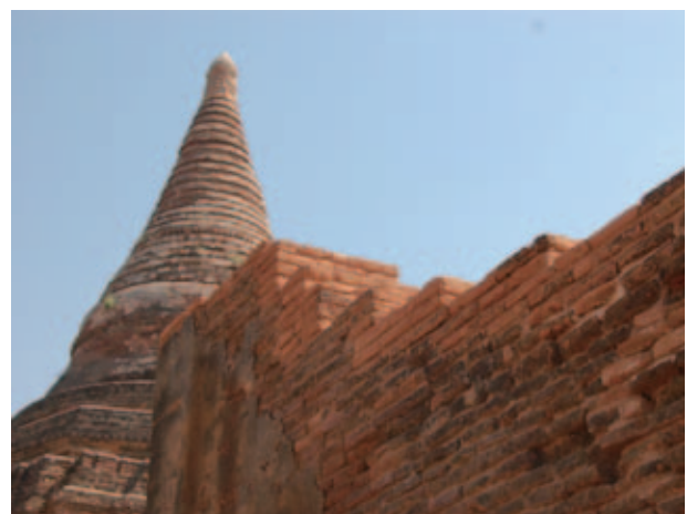
Fig.22 Close-up view of the top of a wall of No. 476
