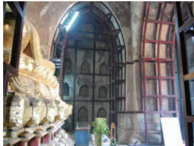
Fig.15 Steel beam supports inside Kyauk-ku-umin
