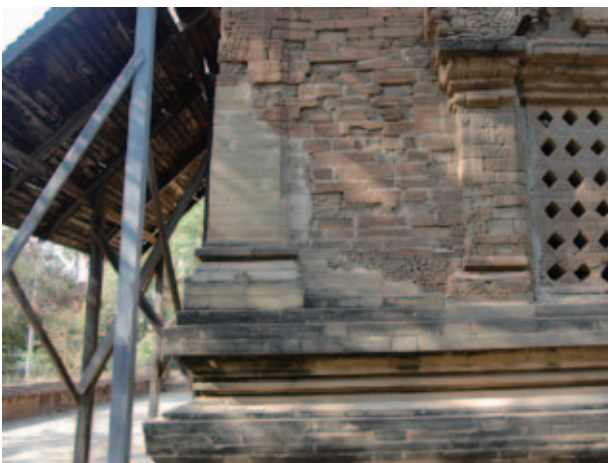
Fig.27 Restored wall corner and temporary roof at Nan-hpaya
