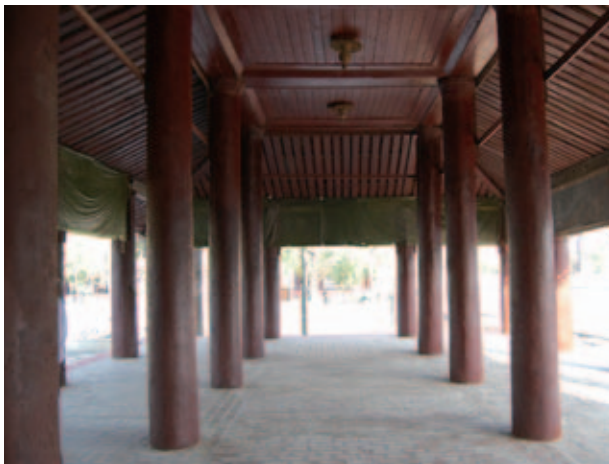
Fig.64 Inside of a zayat building (the pillars are slightly tilted to the left)
