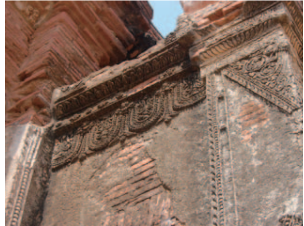
Fig.18 Stucco decoration at the top of a wall at Thambula-hpaya
