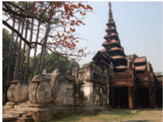
Fig.77 External view of the east façade of Bagaya Monastery
