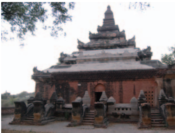
Fig.39 External view of the east façade of Pitakat-taik
