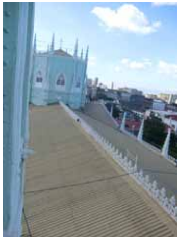
Fig.66 Steel-frame roof of Basilica Minore de San Sebastian
