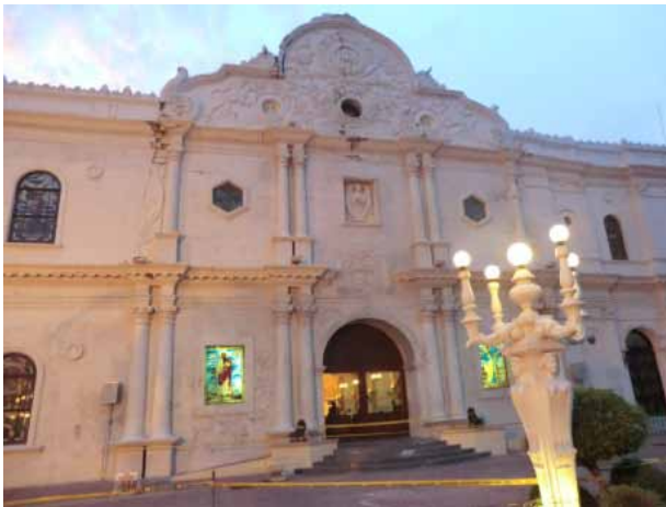
Fig.90 Crack in façade of Cebu Metropolitan Cathedral after earthquake
