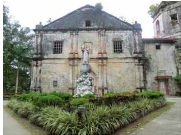
Fig.119 External view of Santa Cruz Church
