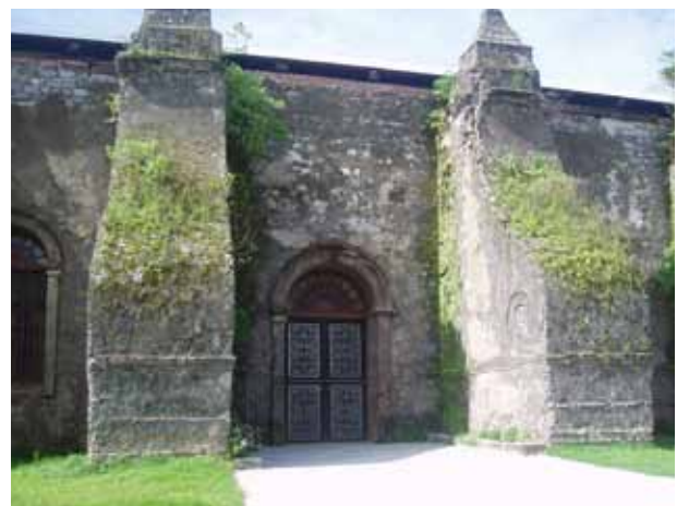
Fig.47 Vegetation on outer wall of San Agustin Church (taken by Juan, in August 2012)
