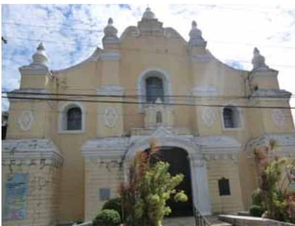
Fig.40 Façade of Santa Lucia Church
