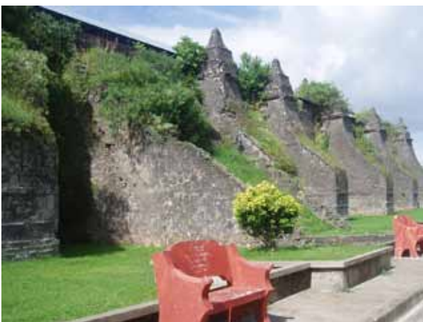
Fig.46 Buttress of San Agustin Church (taken by Juan, in August 2012)
