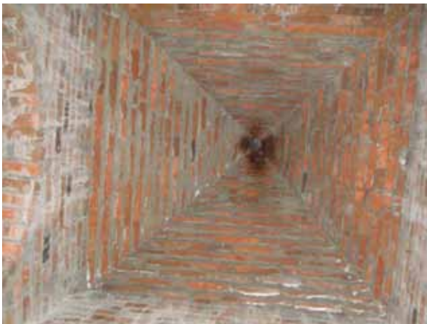
Fig.23 Inner view of belfry roof
