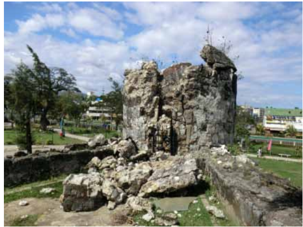
Fig.83 Fort San Pedro after earthquake
