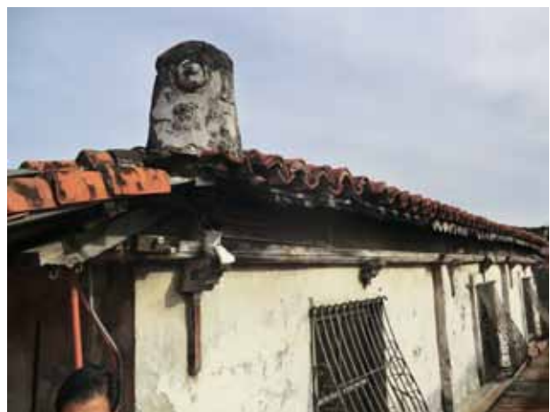
Fig.81 Clay-tile roof of Jesuit House
