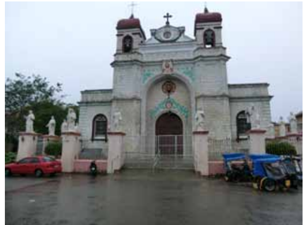
Fig.95 External view of Church of Santa Catalina de Alejandria
