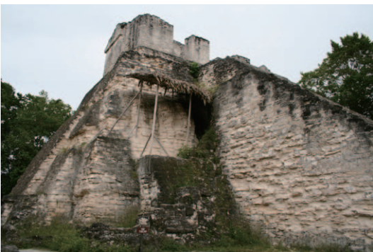
▲ Structure 5D-22 in the North Acropolis, showing the state of erosion and dissolution
