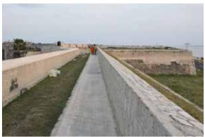
Fig. 53 Upper part of outer wall of the fort after restoration
