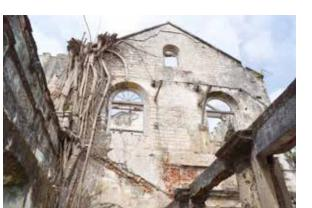
Fig. 18 Damage caused by plant growth
