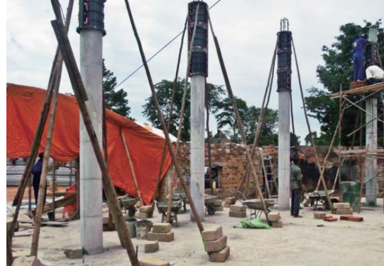
Construction of concrete poles
