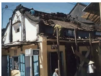
Construction work to replace leaking roofs
