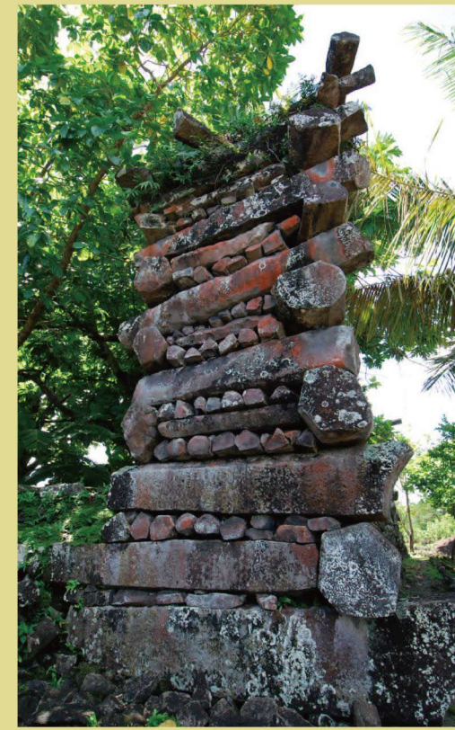
Entrance in the outer wall of Nandauwas. The wall is built of prismatic basalt piled in alternating header-stretcher courses, and rises to a height of approx. 8 m.
