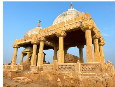
(b) West side (slightly damaged)
