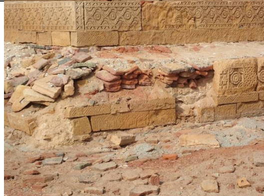
Fig.2 The basement is brickwork, as evidenced by the collapsed sections.
