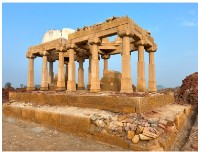
(a) East side(Major damage)
