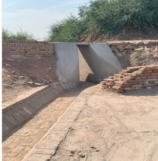
Fig. 4 These photographs were taken at the S.D. and HR area, which depicts the new and old paved/concrete pathway for deep and shallow drainage systems to ease the water flow away from the main structures.
