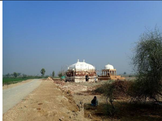
Fig.5 The mausoleum on the right side of the photo was restored after the dome collapsed due to the 2022 flood.
