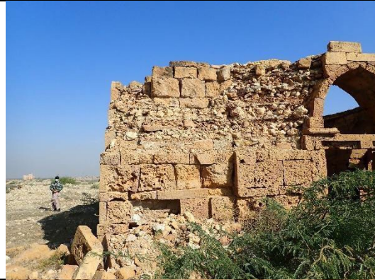
Fig.5 Structure of the stonework. The structure was revealed when a collapse exposed the inner of the walls.
