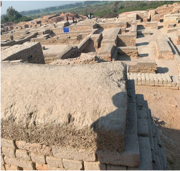
Fig.5 Mud slurry and mud capping works to protect the ruins (i.e. wall and stupa dome) from extreme climatic/weather conditions.
