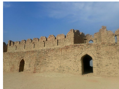
(b) East side (slightly damaged)
