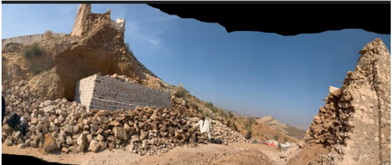
Fig. 2 Collapse of the Shah-Pere Gate and status of reconstruction
