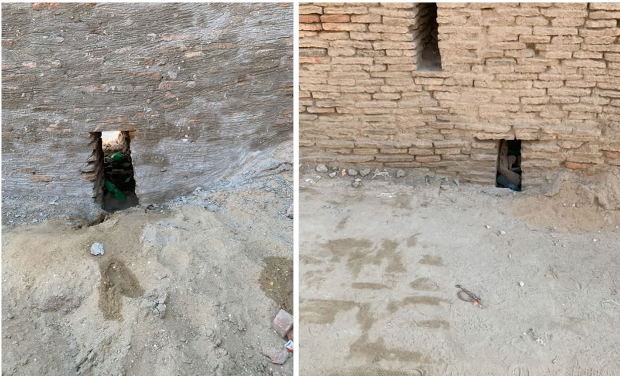
Fig. 7 The existing conditions of the drainage system
