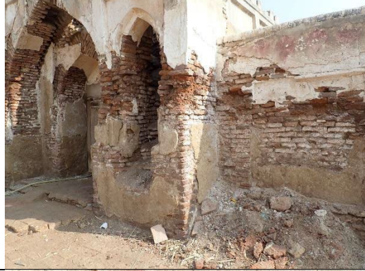
Fig.5 Basic wall structure. The brick wall body is coated with mud and then plastered over.
