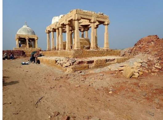
Fig.1 The basic structure of the mausoleum, with a two-tiered platform. The basement decoration, pillars, beams, and dome are made of sandstone.
