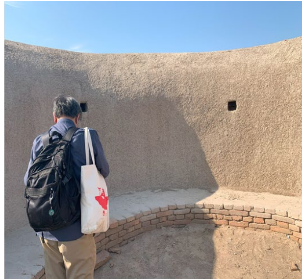
Fig.5 Mud slurry and mud capping works to protect the ruins (i.e. wall and stupa dome) from extreme climatic/weather conditions.
